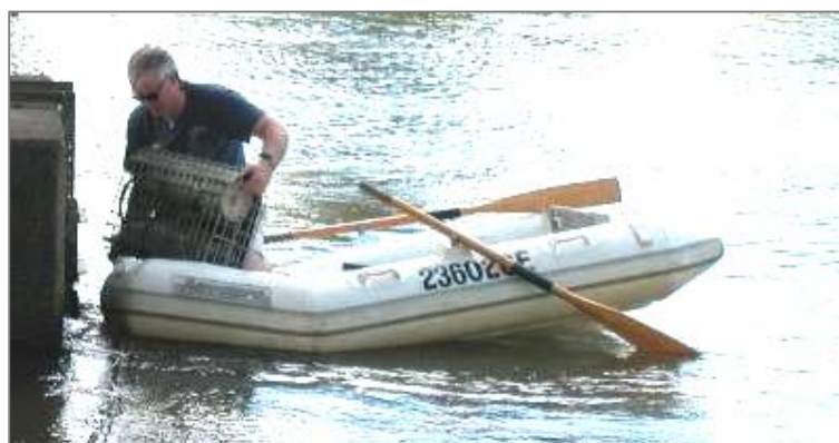
Figure 2 Fitting river logger (in protective cage) to structure on river bridge.
