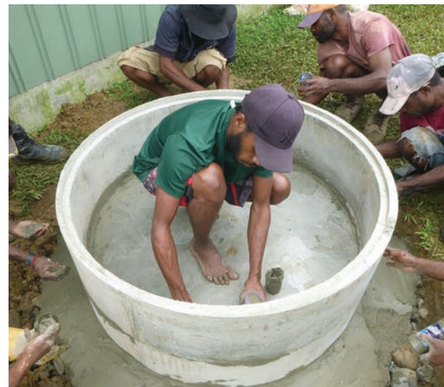
Nuku trainees assemble tank rings. Photos: INLOC
